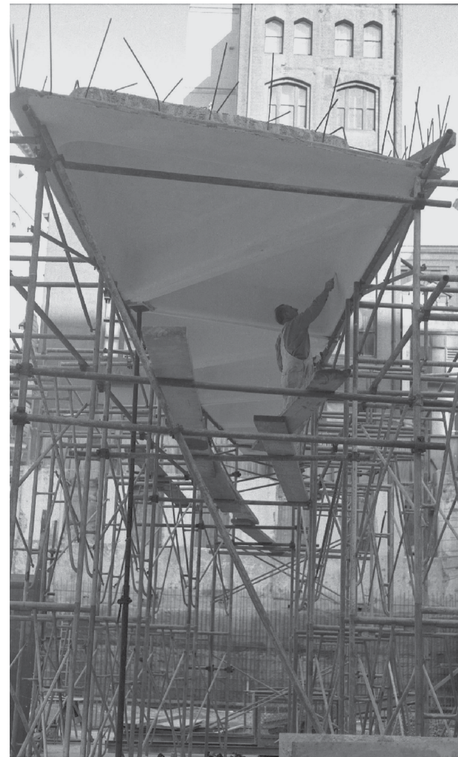
Solaio in ferrocemento / Ferro-cement ceiling 1965 Mockup Australia Square, Sydney, Australia Design Pier Luigi Nervi
