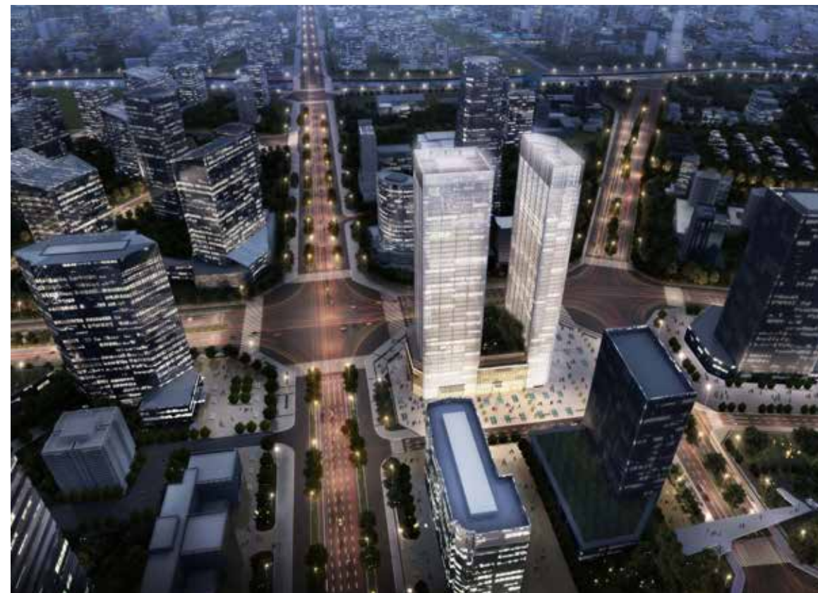
Tonino Lamborghini Center, Chengdu, China In costruzione - 2021 / Under Construction - 2021 Design Studio Marco Piva + JHM
